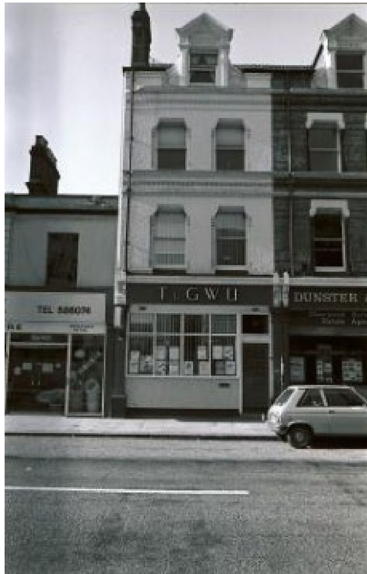
King's Road, Reading, c. 1983. The south side. No. 36 (office of the Transport and General Workers' Union, with "T. & G. W. U." on the fascia, and part of No. 34 (Dunster and Morton, estate agents). 1980-1989: photograph by Terry Allsop (from the Reading Library's Online Archive)
