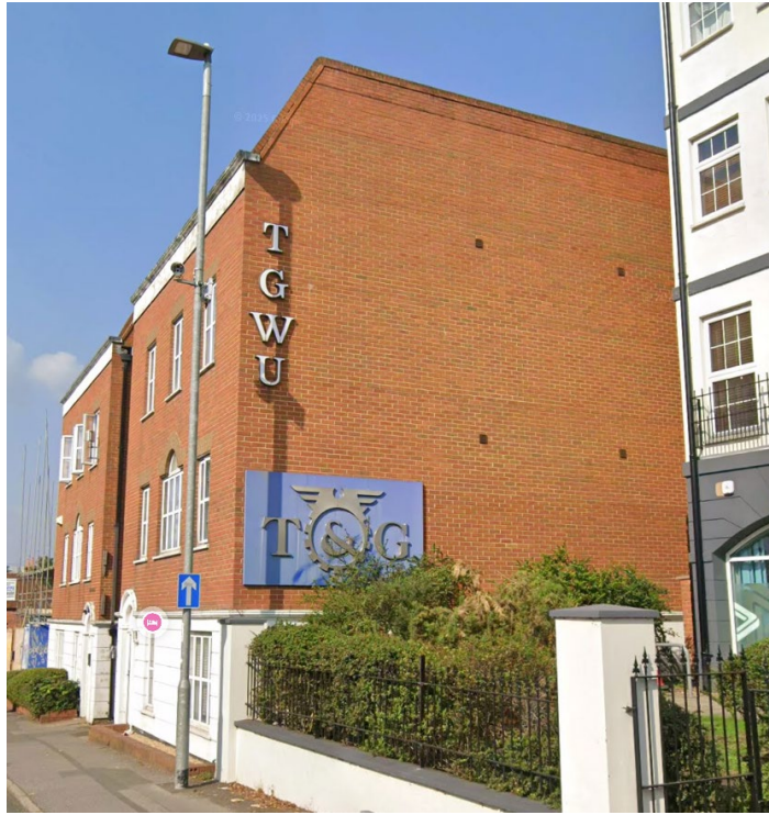
The nominated TGWU Signage at 89 Southampton Street (image is from Google Street View)
